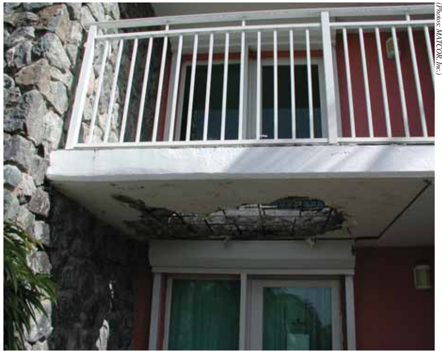
Figure 1: Condominiums along the coast of Florida face serious corrosion issues if not properly protected.
