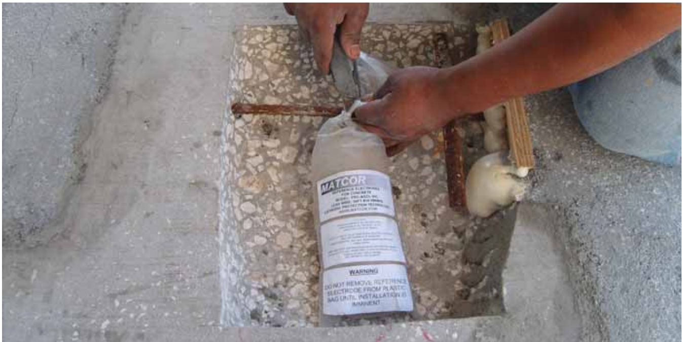
Figure 3: Reference electrode going into concrete repair patch.
