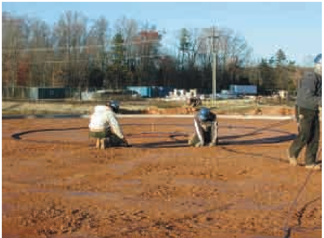
Installation of concentric Matcor SPL-FBR anode rings
