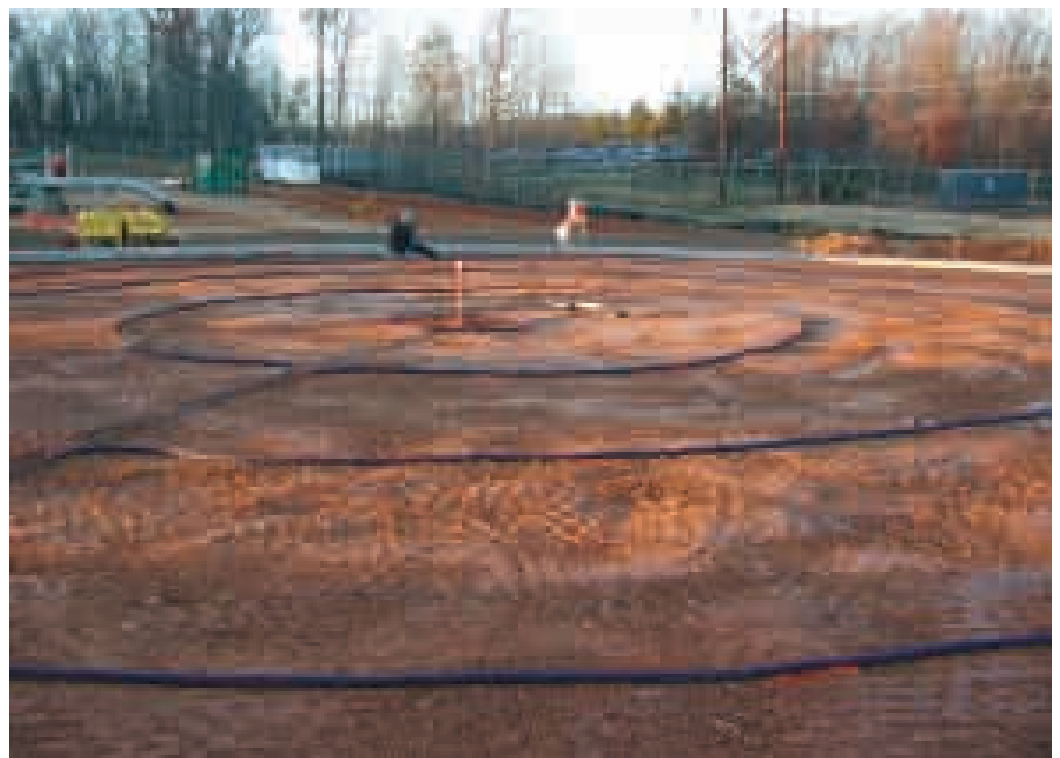
Completed installation of anode rings prior to backfilling
