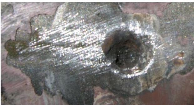
Figure 1. AC induced corrosion.
