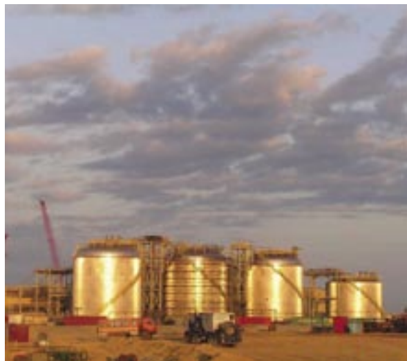
The MATCOR SPL™-Anode System protects tank bottoms and buried piping
