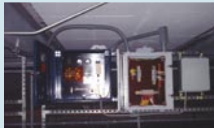
After: With the roof clear of damage, the customized MATCOR CPBD system now protects the VAB roof.
