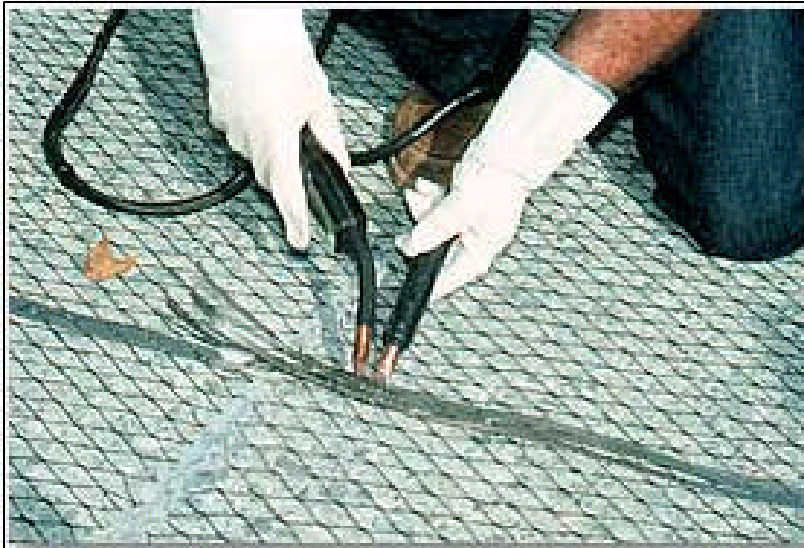
Figure 1 Welding of Titanium Conductor Bar to mixed metal oxide mesh being applied as an overlay
