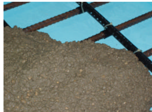
Figure 3 SPL™-HDPE Anode with snap in place insulators
