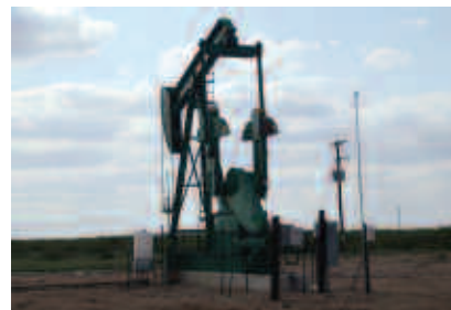
The Sprayberry Field has more than 4,000 bores; at least a quarter of them are protected by MATCOR Mini-Deep™-Anode Systems.
