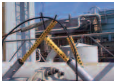
Driving anodes and reference cells being driven to depths of 40 feet for LNG tank piling systems.
