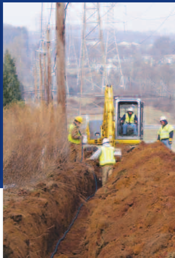
The MITIGATOR™ being installed along a HVAC corridor.
