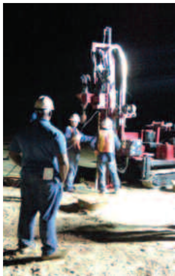
Driving anodes and reference cells being driven to depths of 40 feet for LNG tank piling systems.
