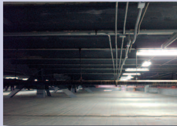
After MATCOR installed a CP system on NASA's 215,000 square foot crumbling Vehicle Assembly Building roof, the concrete crumbling and deterioration stopped.
