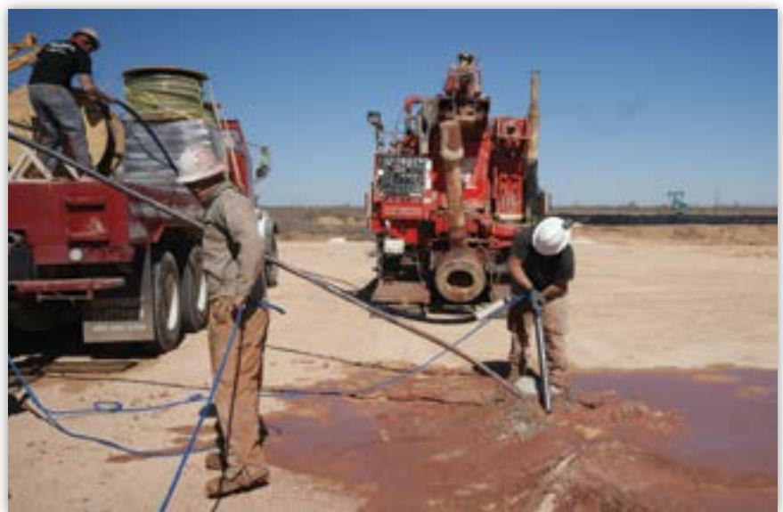
The Durammo™ Deep Anode System installed to protect oil wells in Texas from corrosion.
