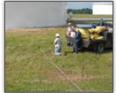
MATCOR Iron Gopher® HDD installation beneath a tank
