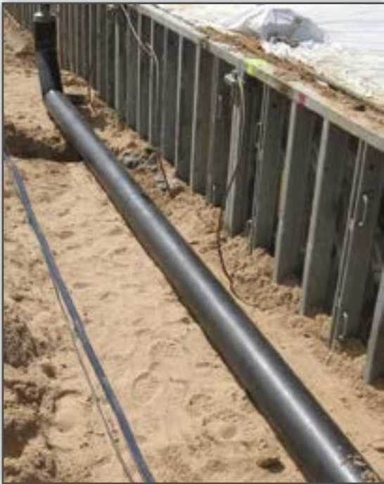
MATCOR SPL-FBR-Anode provides cathodic protection for power company assets
