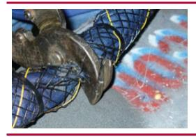
**3.** Using an appropriate sized cutting tool, cut completely through the entire assembly including the anode and internal header cable yielding two separate pieces.
