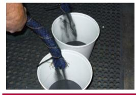
**4**. Carefully pour coke backfill from each end to approximately 10 cm (4") of length. Dispose of coke backfill in accordance with acceptable site regulations and requirements.
