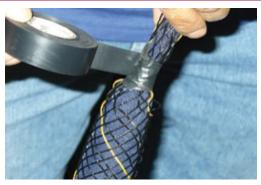
**6**. Using electrical tape, secure the tightly packed coke to the internal header cable and anode assembly.
