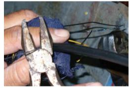
8. Trim the exposed anode wire back as close as possible to the end of the SPL–FBR Linear Anode.
