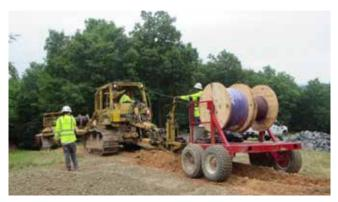
Figure 3. Cable plow installation of linear anode to the side of the pipeline along the ROW.
