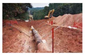
Figure 2. Recoating operation along the open right-of-way (ROW).
