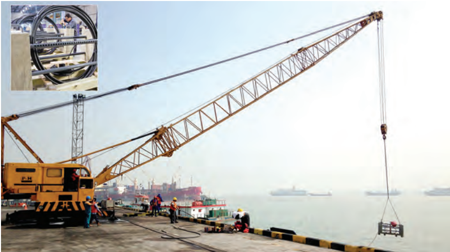
FIGURE 2 Anode sled installation.
