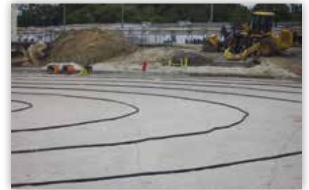
MATCOR Tank Ring SPL-Anode installation
