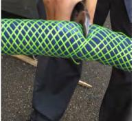
• Use the cutting tools to cut completely through the Mitigator braiding, fabric housing, Powerfill (see #3 for instructions on preserving the Powerfill) and internal copper wire to yield two pieces.
