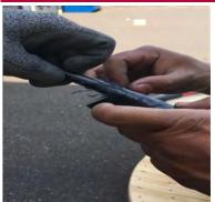
8. Gather the cut ends of the fabric and braiding securely over the connection you have just created. Wrap with electrical tape to secure the Powerfill in the sock and to clean up the ends.
