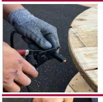
**1**. Use the cable stripper to remove about 2" of vinyl jacket from the #2 HMWPE cable, exposing bare copper wire.
