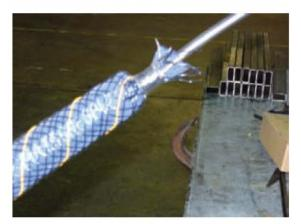
Install anode segment in accordance with the design/installation requirements.
