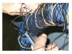
Using a knife, carefully trim away excess braiding materials and inert fabric housing. Take care not to damage or cut the insulation of the internal header cable while removing the excess materials.
