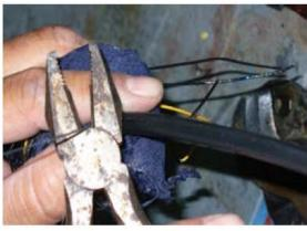
Trim the exposed anode wire back as close as possible to the end of the  $SPL^{TM}$ -FBR Linear Anode.
