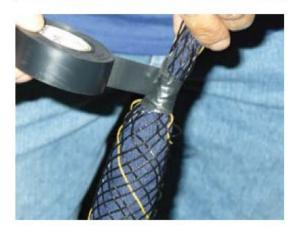
6 Using electrical tape, secure the tightly packed coke to the internal header cable and anode assembly.
