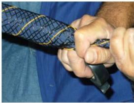
Tightly compress the coke backfill around the internal header cable and anode assembly.
