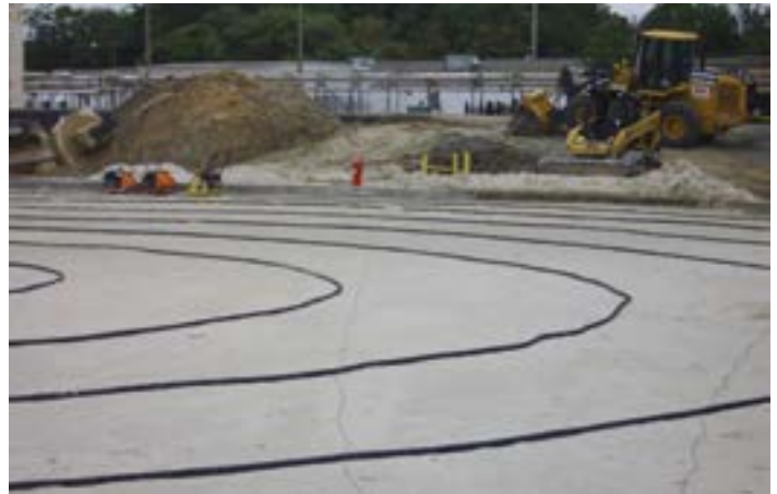
MATCOR Tank Ring SPL-Anode Installation
