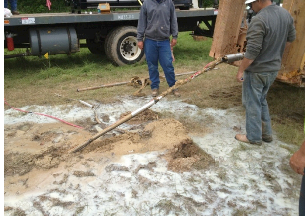
Figure 2 - Gopher exiting the borehole after completion of pulling operation.
