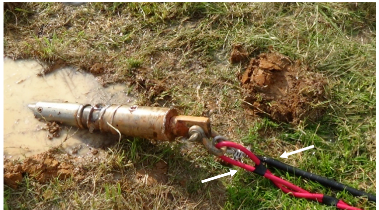
Figure 1 - Gopher and auxiliary anode header cable (red) attached to drill pipe prior to pulling through bore hole.
