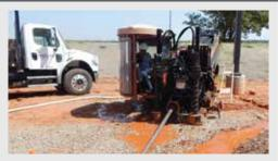
MATCOR products and services protect infrastructure assets from corrosion. Shown above is one of our HDD rigs installing MATCOR SPL<sup>TM</sup>-Anodes to protect aboveground storage tanks.
