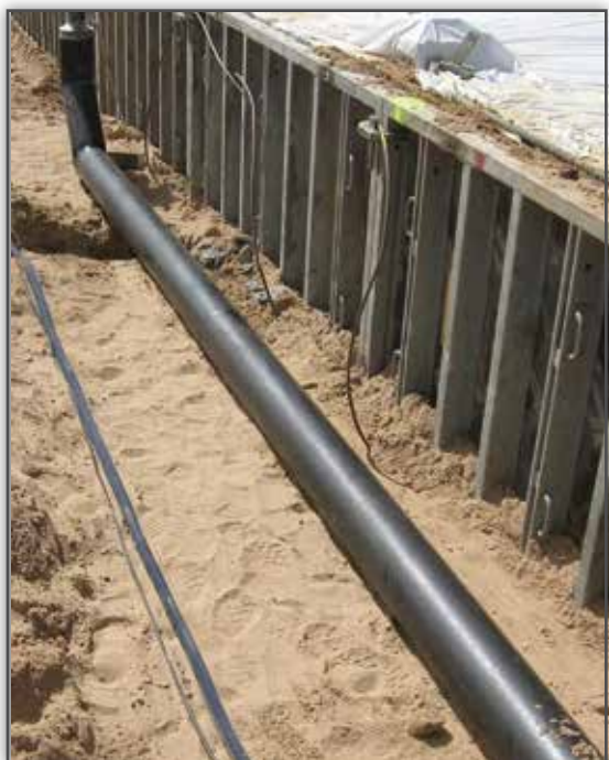
MATCOR SPL-FBR-Anode provides cathodic protection for power company assets
