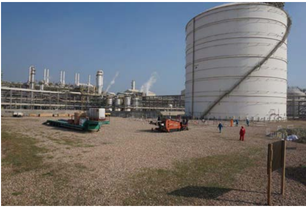
Figure 4. HDD drill rig and support equipment preparing for installation.
