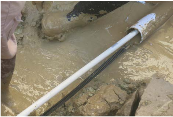
Figure 1. Anode and vent pipe assembly being installed in bore hole.
