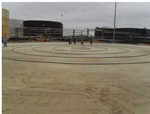
Figure 3. Typical anode installation: concentric ring impressed current CP anodes being installed.
