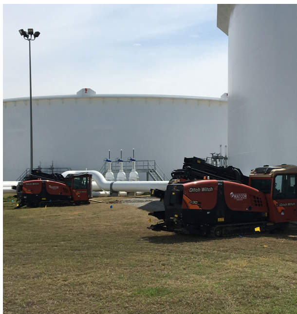
Figure 2. HDD drills boring under an existing tank to install new anodes.
