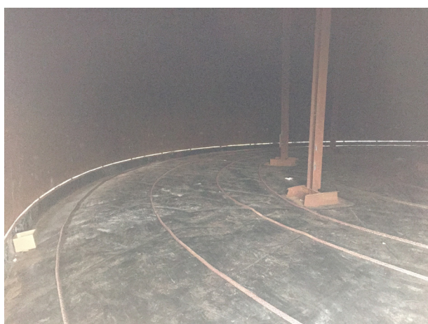
Figure 1. Concentric ring linear anode being installed on top of liner in a tank bottom replacement project.
