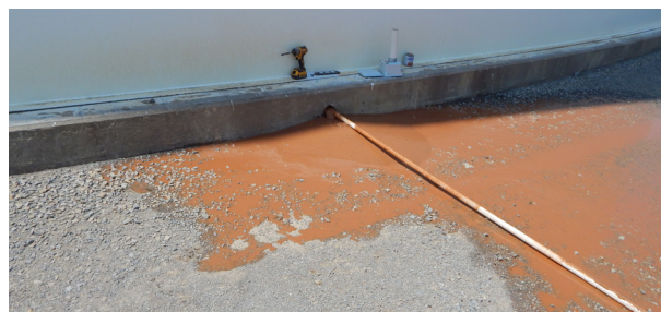
Figure 3. Hydrojet anode installation using a core drilled hole through the ring wall.
