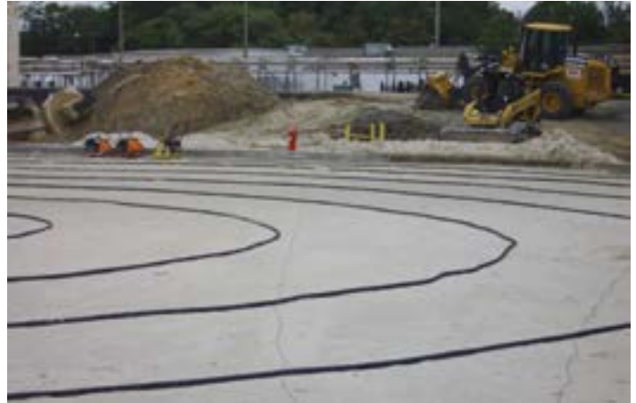
MATCOR Tank Ring SPL-Anode Installation
