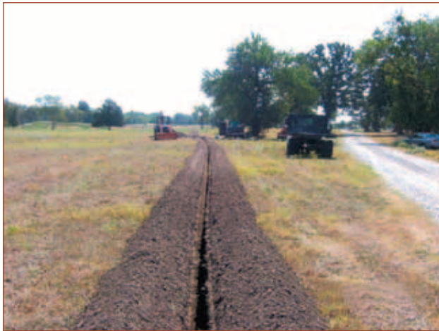
Figure 2. MATCOR SPL™-FBR linear anode installation using a trench unit.
